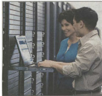
Computing needs: Support will be from the National Grid service providers
